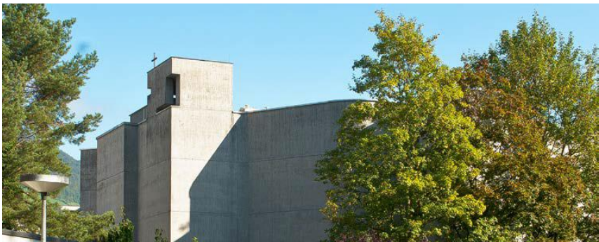
Exterior view of the convent church, Ingenbohl
