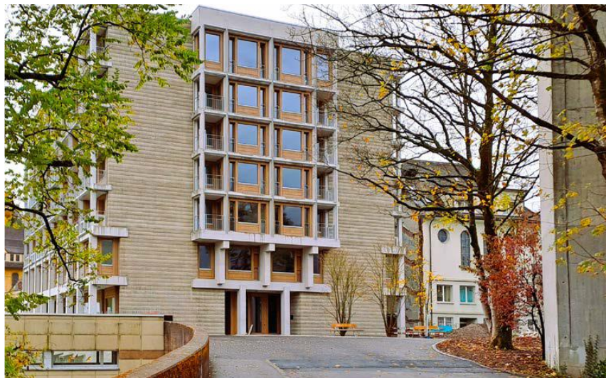
St. Joseph nursing home, access road
