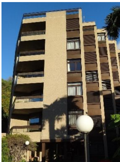
Former school Villa Erica
