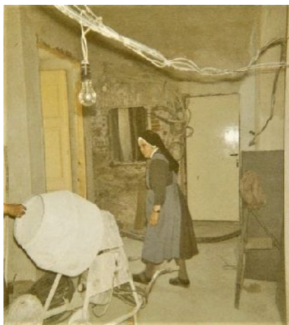
Cerová during the renovation
